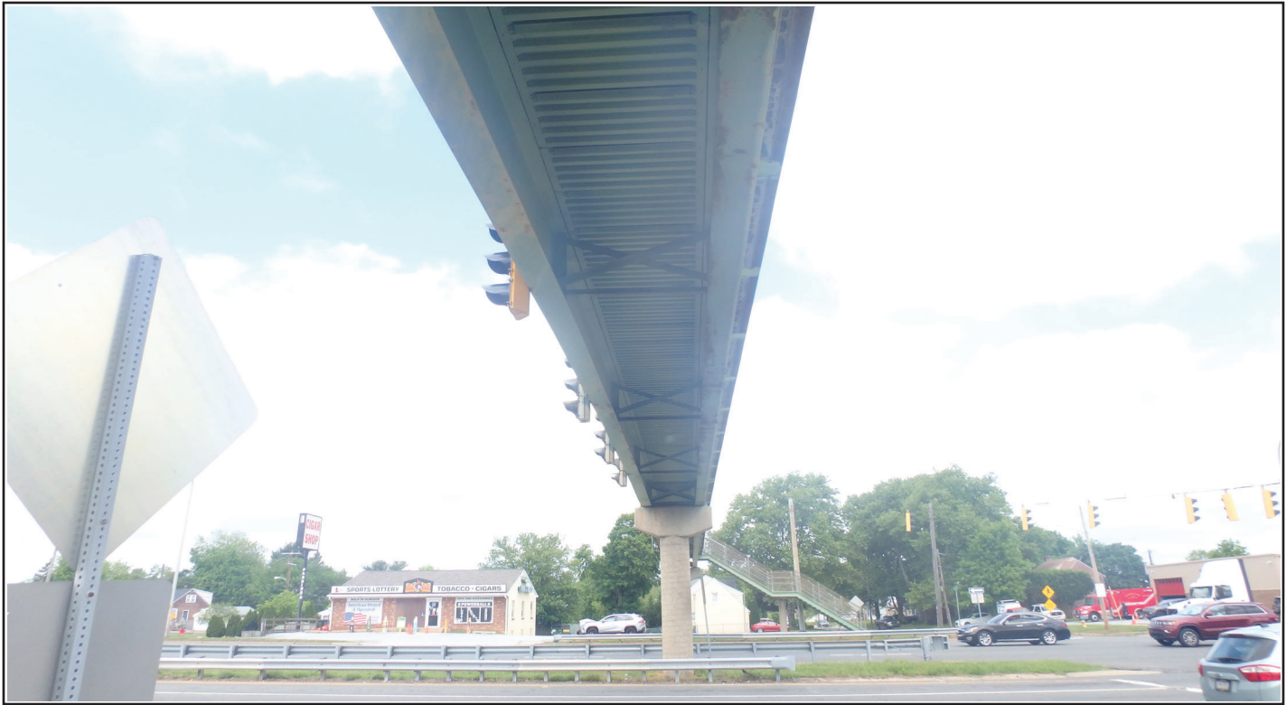
3 SP.1 GENERAL VIEW LOOKING WEST
