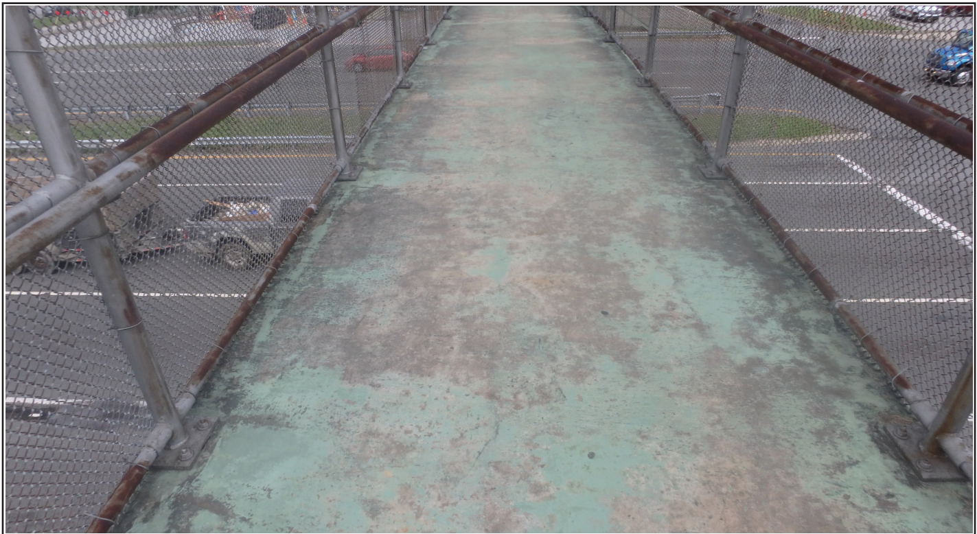
6 SP.1 DECK VIEW LOOKING WEST
